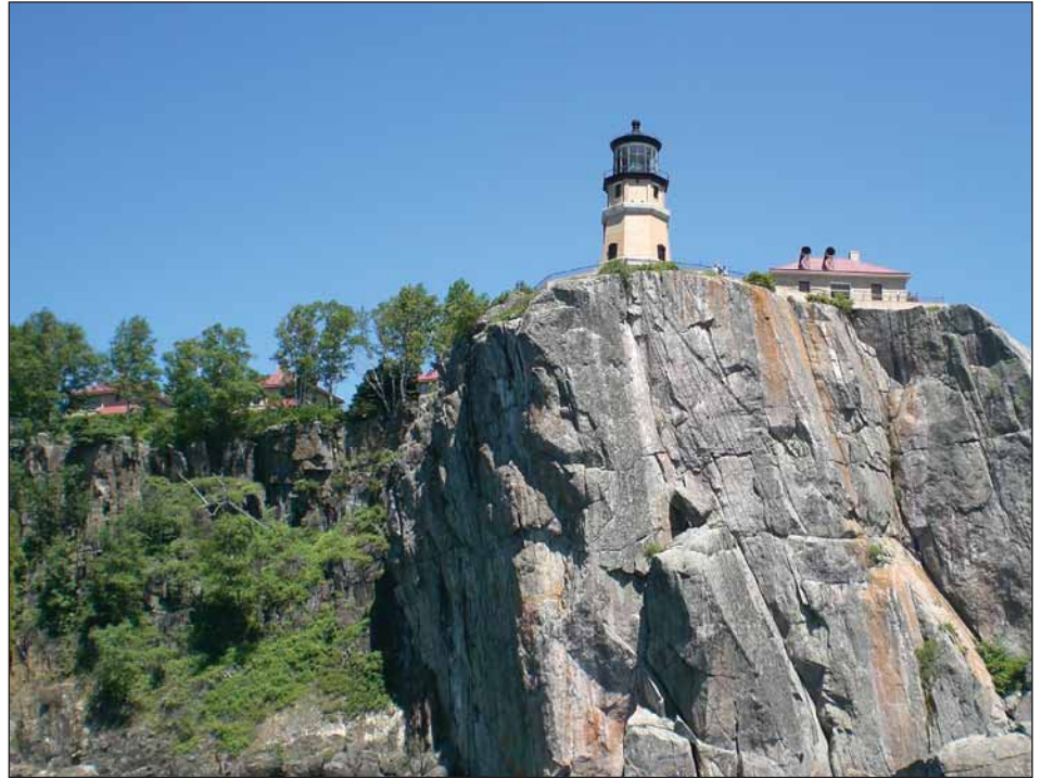
Split Rock Lighthouse.
